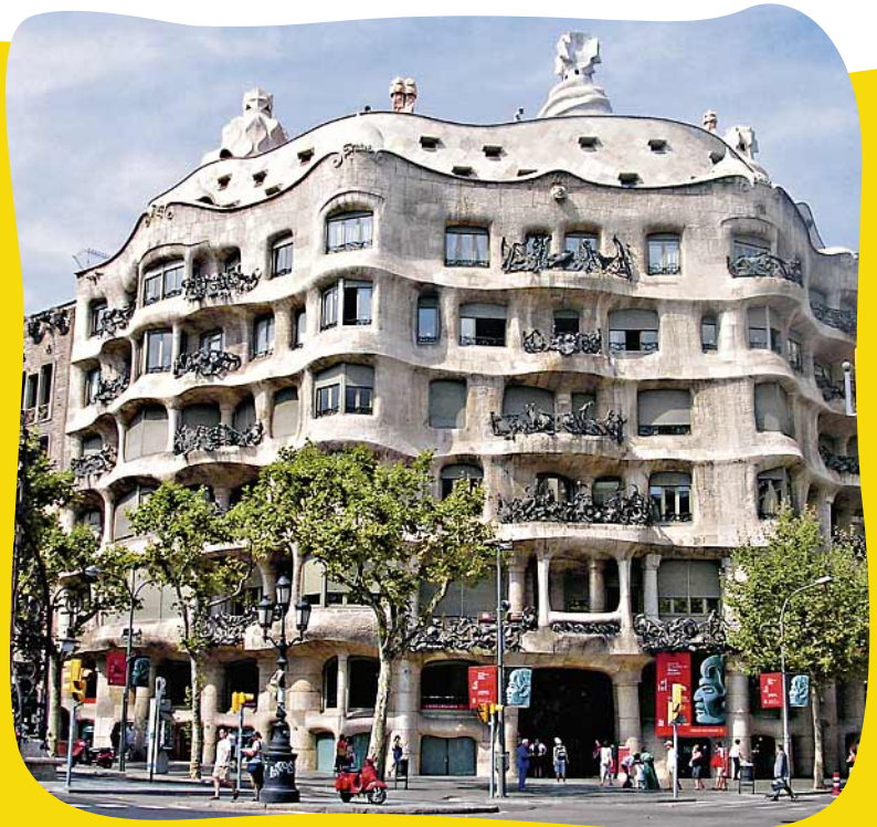
In the Casa Milà (1906–10) natural ventilation makes air conditioning unnecessary.
